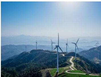
Energy and Power
